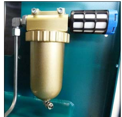
Oil / water separators final stage
