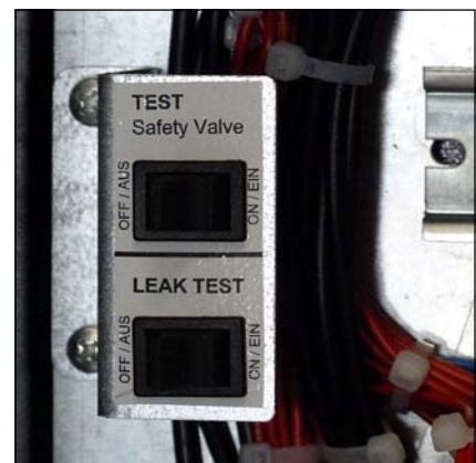
Leak test switch (lower)
