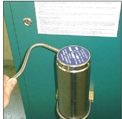
Fig. 1 - Unscrew the filter housing cover.
